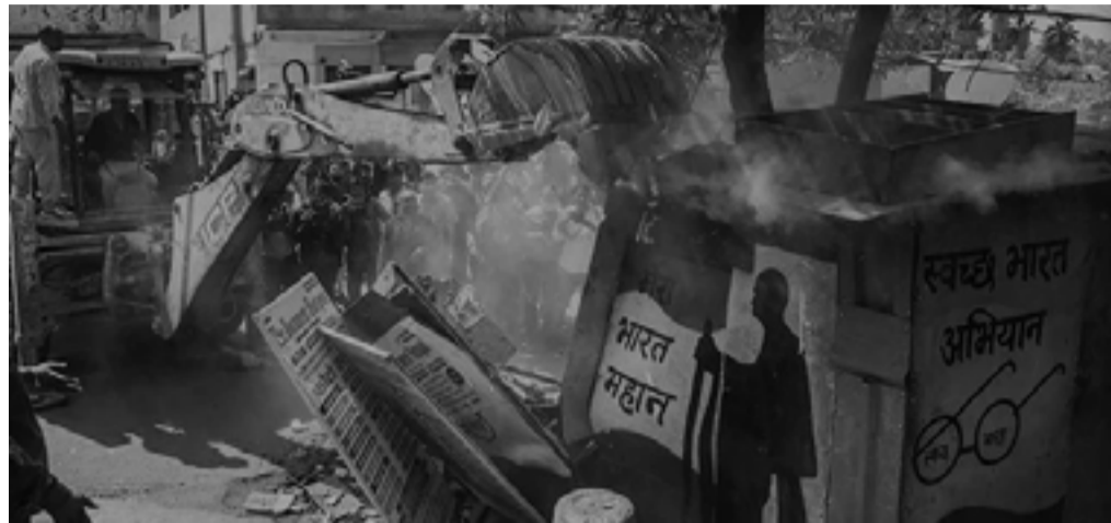
Bulldozer demolishing the shop at Jahangirpuri, New Delhi
